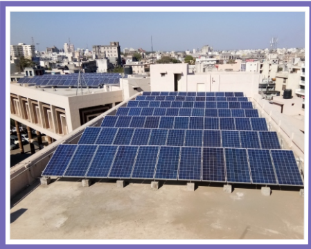
Solar Panel Structure Mounting on RCC
