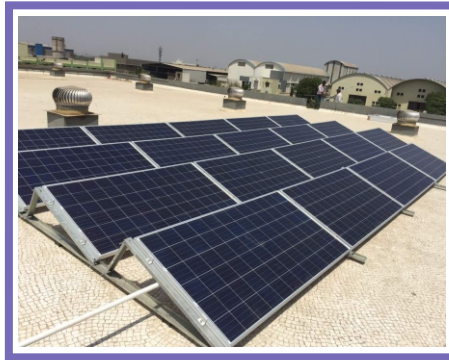
Solar Panel Structure Mounting on RCC
