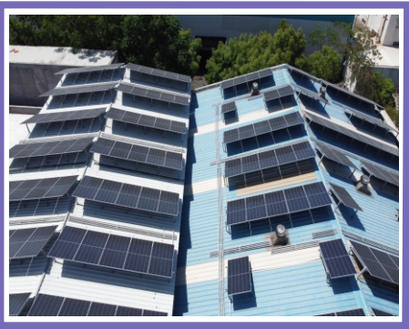
Solar Panel Structure Mounting on Tin Shed
