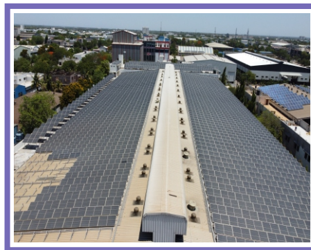
Solar Panel Structure Mounting on Tin Shed
